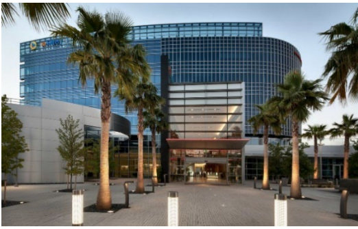
Photo of the CA Lottery Building's exterior.
